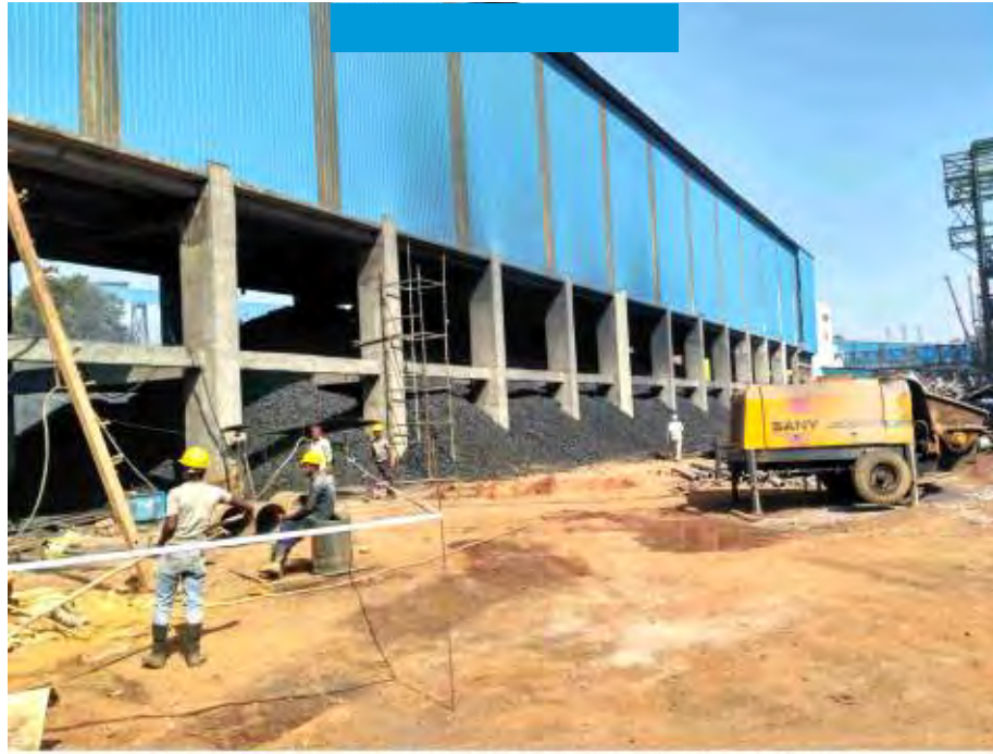
Emergency coke storage yard made operational Bhilai Project
