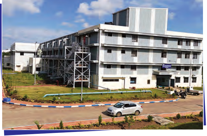
HAL NASIK PROJECT- MAA BUILDING
