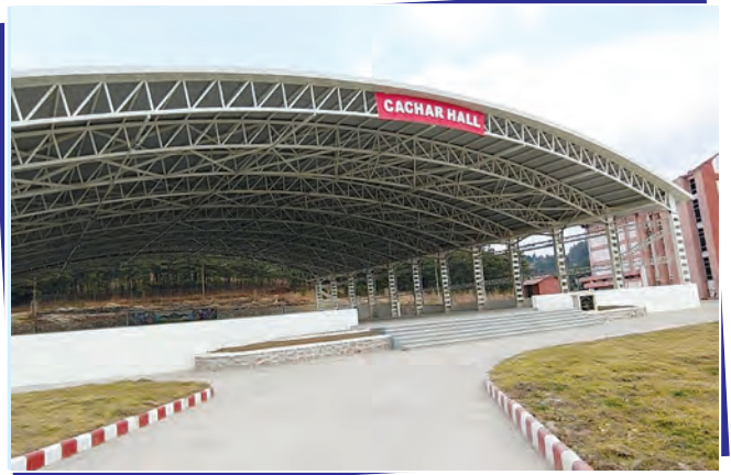
TRAINING SHED, LAITKOR, SHILLONG
