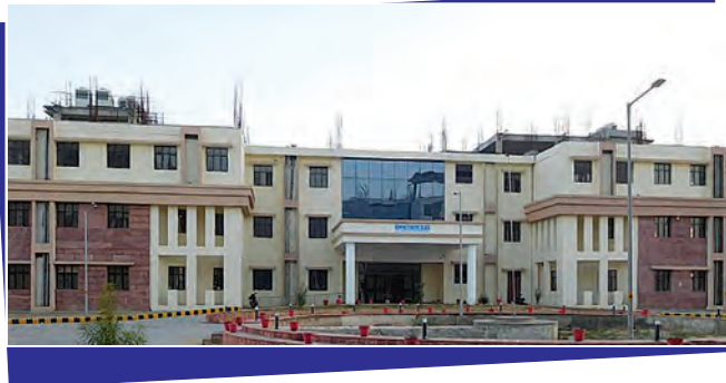
Admin Block, Barmer Medical College, Rajasthan
