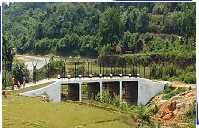
BOX CULVERT, ROAD & FENCE, TRIPURA
