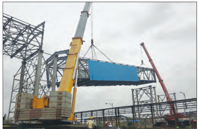
Bhilai Steel Plant Project- Conveyor Gallery Erection over Rail Line
