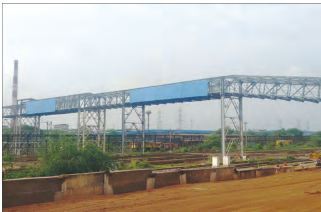
Bhilai Steel Plant Project- Conveyor Gallery Erection over Rail Line
