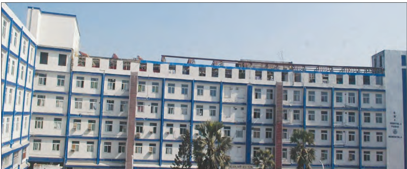
ESIC Hospital Project, Maniktala, Kolkata
