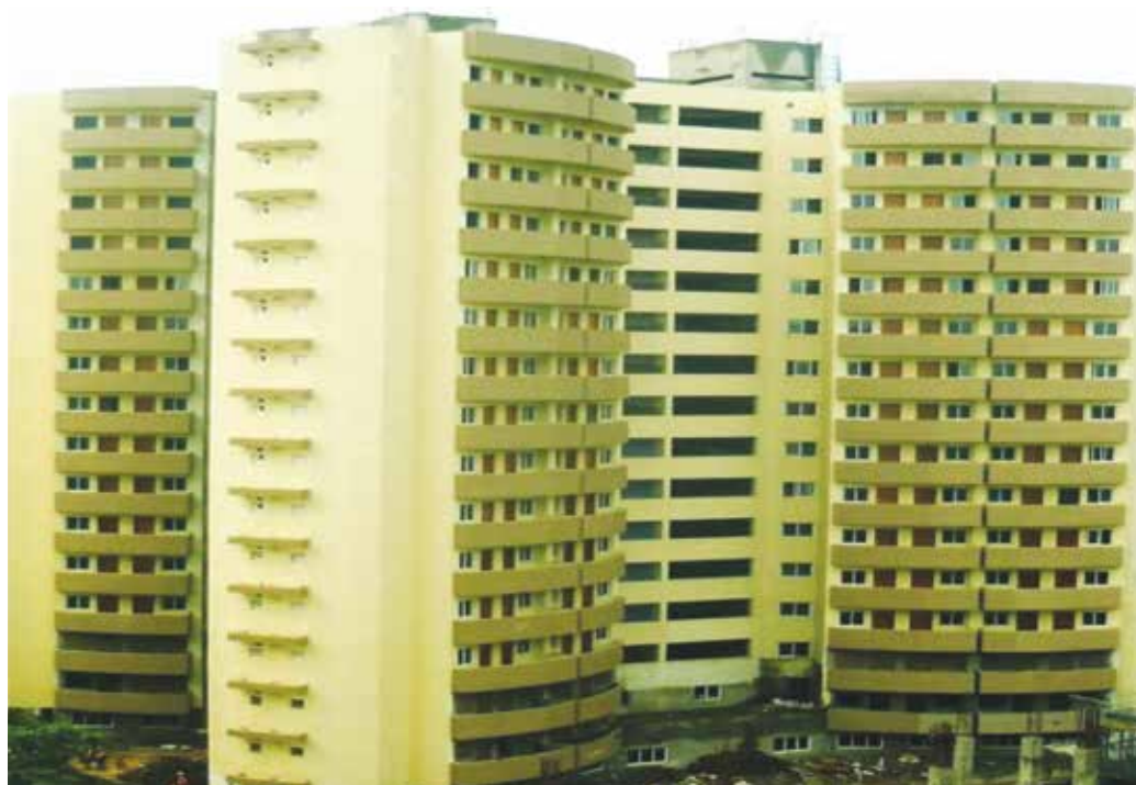
ESIC Project, Joka, Kolkata - New Hostel Building
