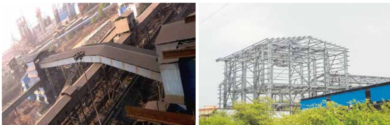
Bhilai Steel Plant- Junction house along with Conveyor Gallery
