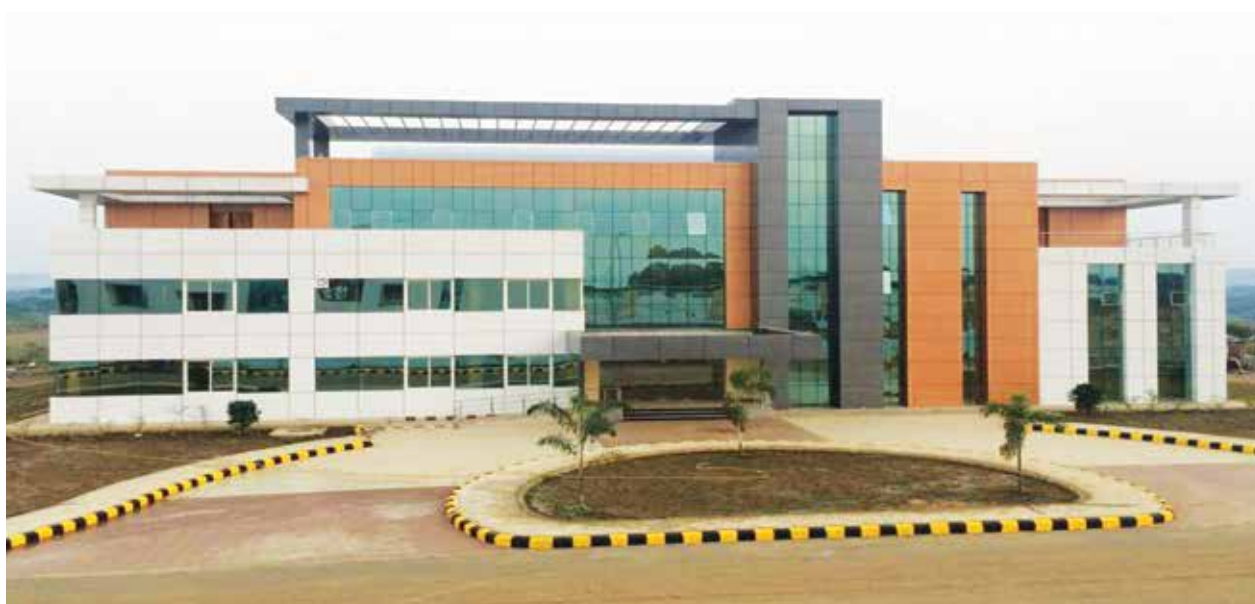
ITBP Jabalpur Project - Administrative Block
