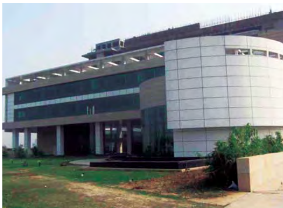
Construction of OIBD Bhawan at NOIDA
