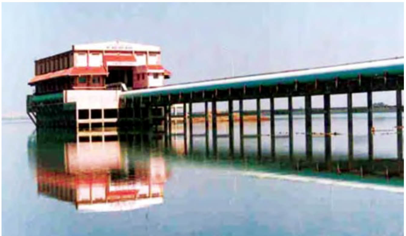
Jackwell – Pumhouse In WSS Project, Nashik
