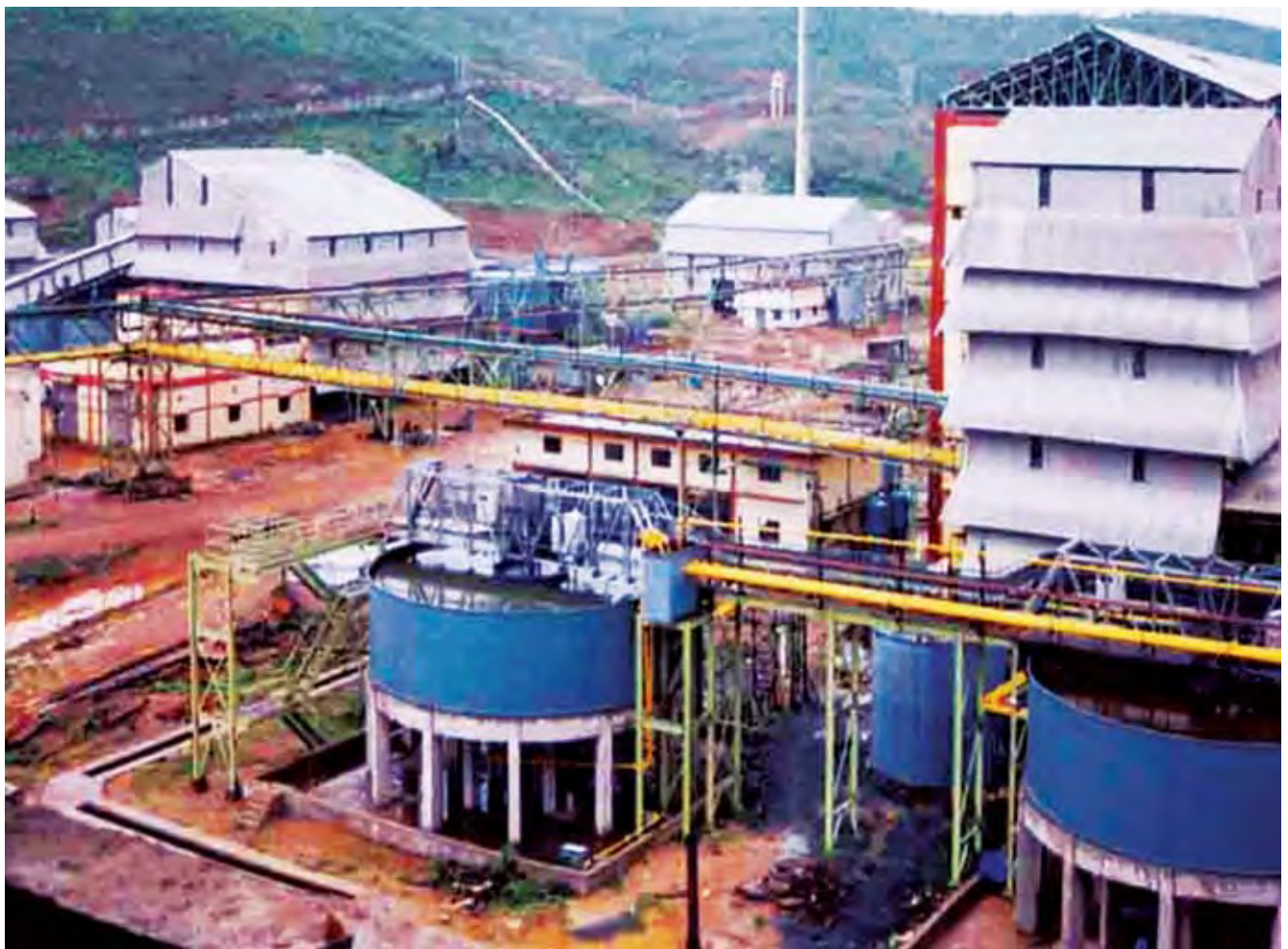
Ore Processing Plant, Jharkhand For UCIL
