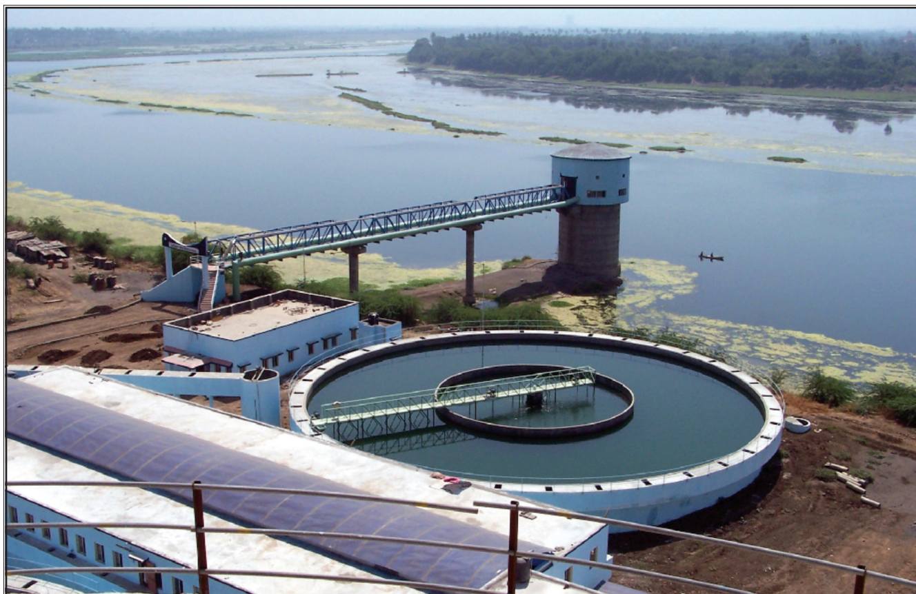
Wss at Variav - View of 10m Dia intake Well in 15m deep riverbed with 14m Dia Pumphouse & 60mld Wtp
